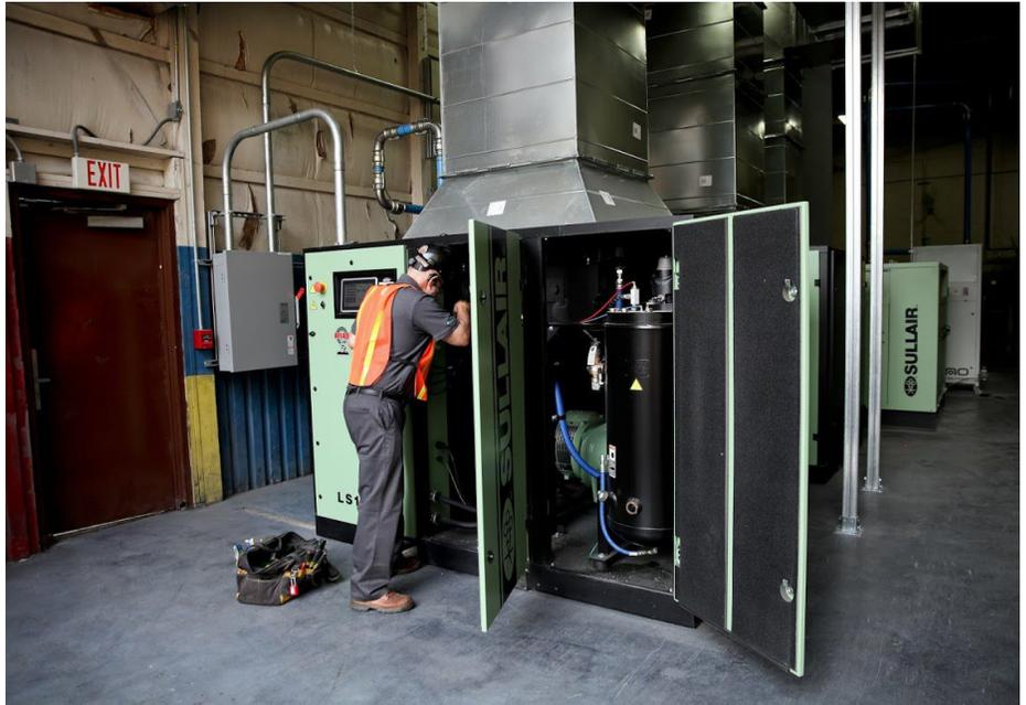
*Atlas Machine & Supply Sullair service technician works on an LS Series compressor*
